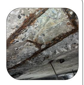
along with the steel rods. All of the areas will be addressed from the underside, eliminating the need for tile work repair if it was to be done from the top.
